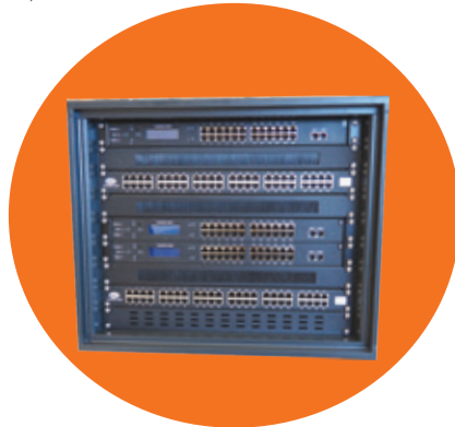
INSTRUMENT ROOM 9U PHONTECH SYSTEM CABINET
